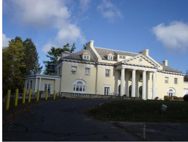
Figure 51. Mansion on Site, (by author)
