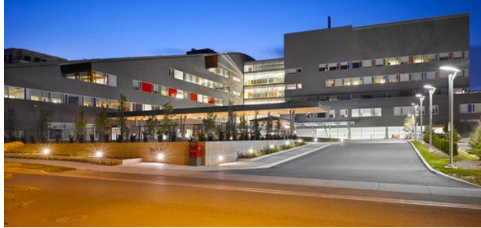
Figure 11. Bloorview Hospital, Canada, Exterior, http://www.metropolismag.com/story/20080220/health-and-happiness
